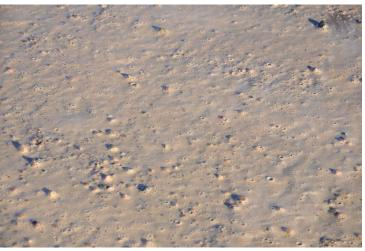
By enhancing liquid magnesium chloride with complex sugars, we have created a product that is ideal for dust control and stabilization on base courses with fewer plastic materials. The additional binding capabilities and deeper color of the CS blends offer a longer lasting road and an aesthetically pleasing surface.
